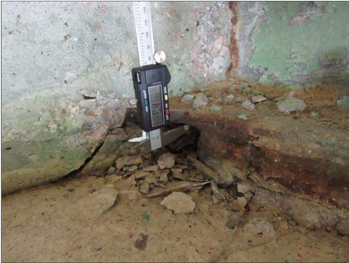
Span 4 Beam 4: 4 INCH LONG X FULL WIDTH CORROSION WITH SECTION LOSS ON LEFT BOTTOM FLANGE AT FAR END, 7/16 INCH THICKNESS REMAINING (PAR)
