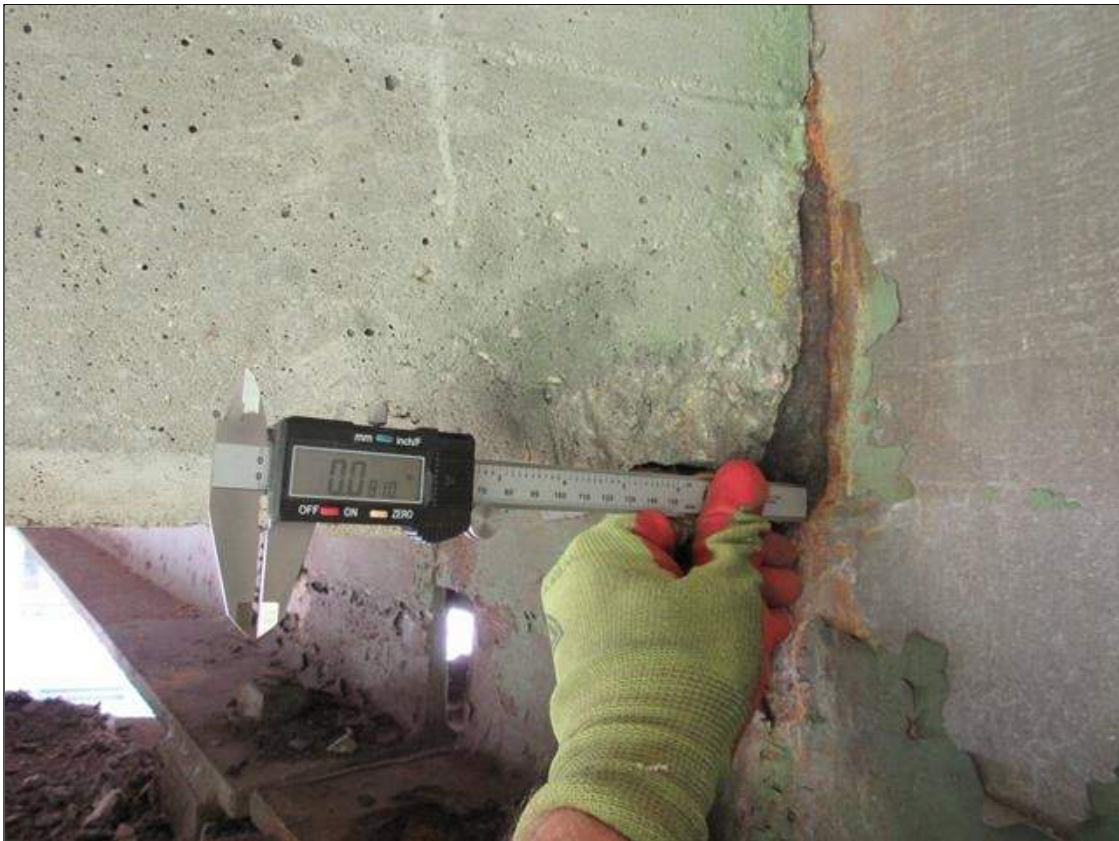
Span 4 Beam 2: ACTIVE CORROSION IN WEB RIGHT SIDE AT NEAR END DIAPHRAGM, 8 INCHES HIGH X 1.25 INCH WIDE WITH 1/16 INCH SECTION LOSS (9/16 INCH REMAINING)
