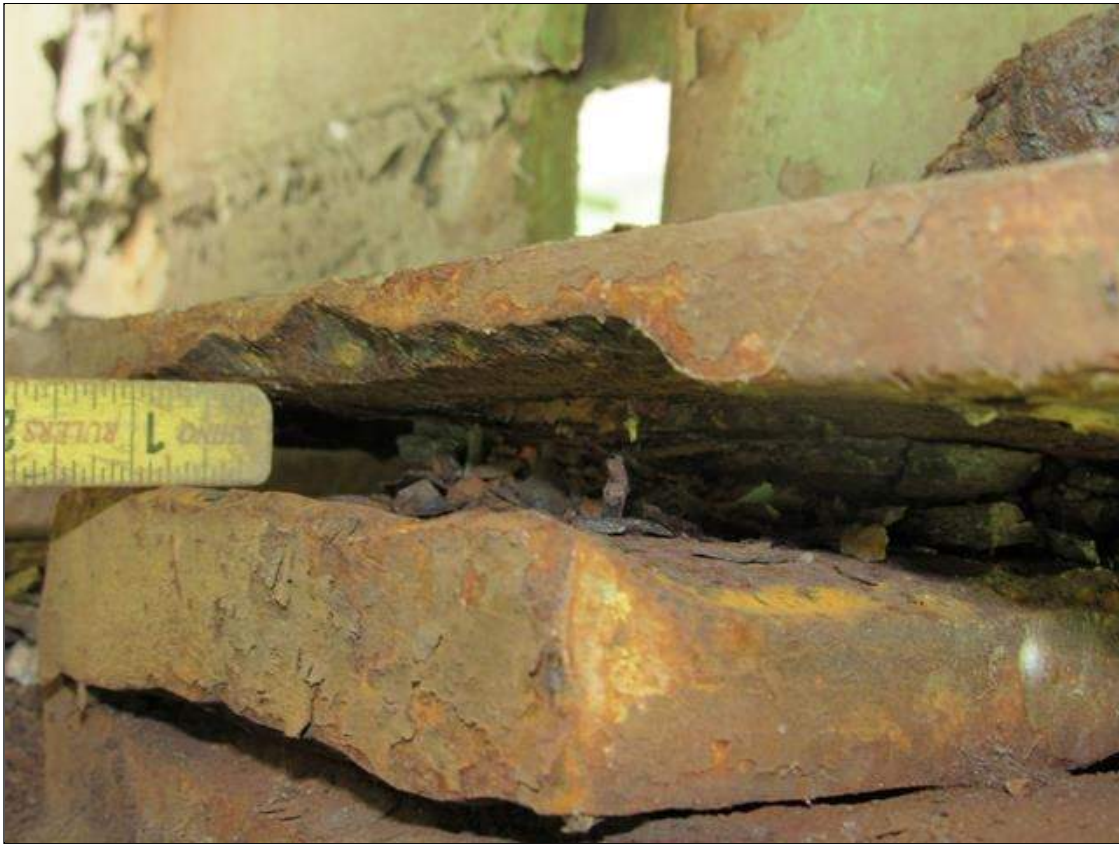
Span 4 Beam 2 - Near Bearing: PAR: 7 INCH LONG X 4 INCH WIDE LOSS OF BEARING AREA UNDER RIGHT BOTTOM FLANGE DUE TO SEVERE CORROSION WITH SECTION LOSS OF BEARING PLATE. RIGHT ANCHOR BOLT IS CORRODED WITH 100 PERCENT SECTION LOSS - NCDOT NOTIFIED 8/13/2022 (PAR)
