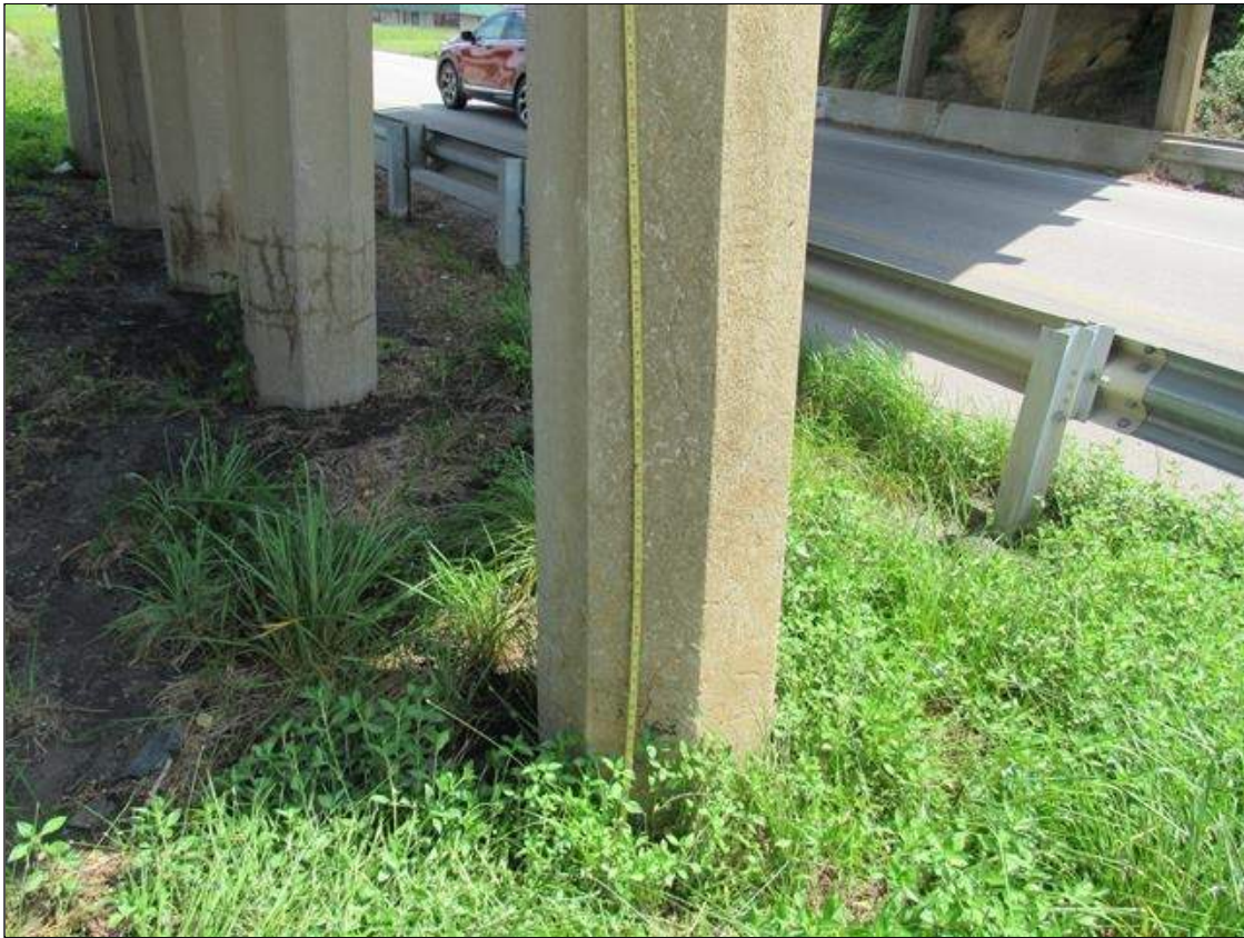
Bent 2 Pile 5: VERTICAL CRACK 8 FEET LONG X UP TO 1/32 INCH WIDE AT SOUTHWEST CORNER EXTENDING UP FROM GROUNDLINE
