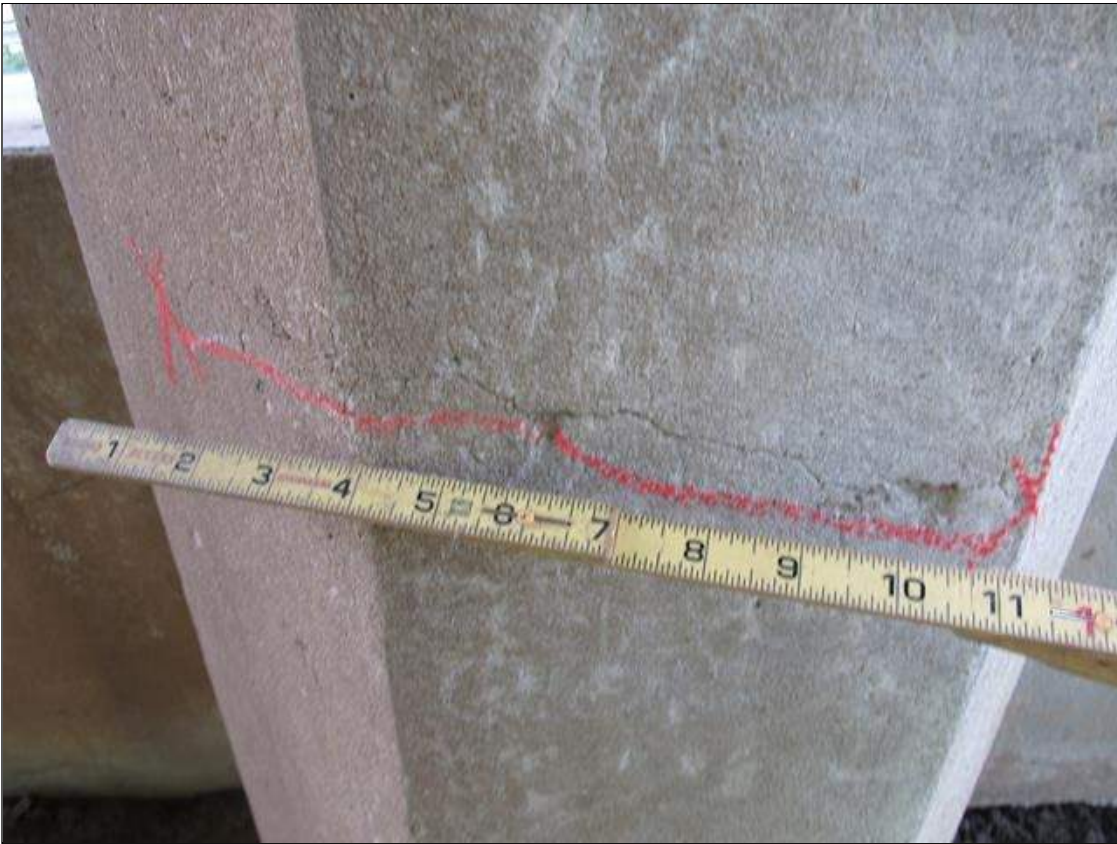
Bent 3 Pile 2: 0.010 INCH WIDE HORIZONTAL CRACK IN EAST FACE, 3 FEET 6 INCHES UP FROM GROUND
