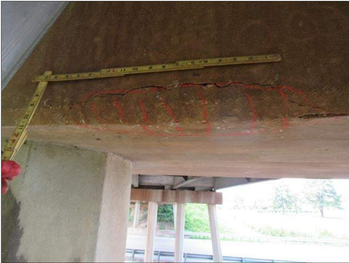
Bent 3 Cap 1: 0.03 INCH WIDE X 18 INCH LONG IN EAST FACE OF CAP ABOVE PILE 3 VERIFIED AT AREA OF DELAMINATION 20 INCHES LONG X 2 INCHES HIGH X 4 INCHES WIDE ON LOWER EDGE
