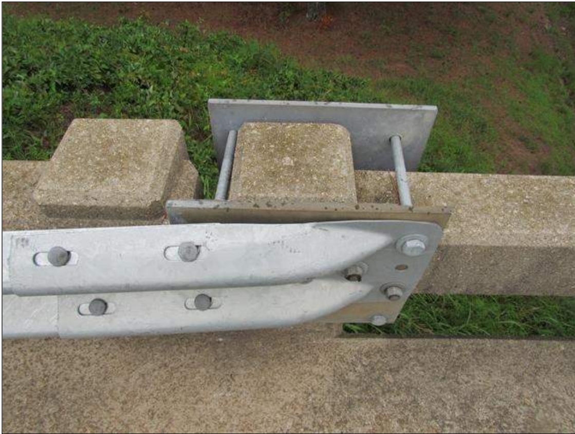
TYPICAL GUARDRAIL ATTACHMENT TO BRIDGE RAIL (SOUTHEAST SHOWN, ALL OTHERS SIMILAR)
