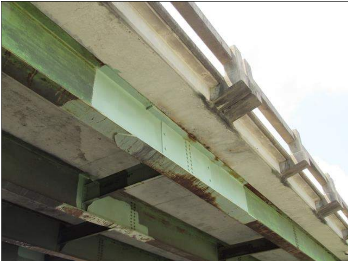
Span 3 Deck: MINOR IMPACT DAMAGE ON UNDERSIDE AT 2ND DIAPHRAGM, LEFT OF BEAM 4 AND BOTH SIDES OF BEAM 1
