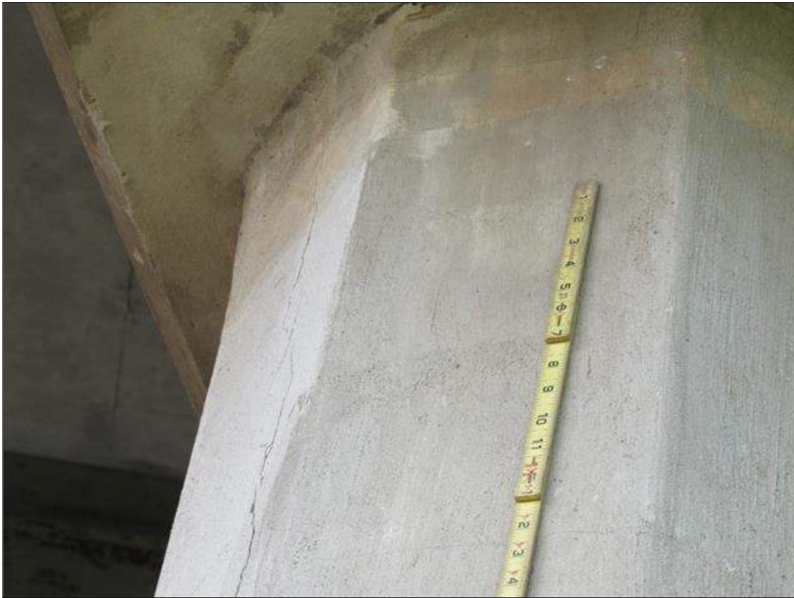
Bent 1 Pile 1: 0.007 INCH WIDE HORIZONTAL CRACK 6 INCH BELOW CAP IN WEST FACE, VERTICAL CRACKS ON NORTHWEST AND NORTHEAST FACES UP TO 0.016 INCH WIDE X 10 FOOT HIGH (SEE PHOTO)
