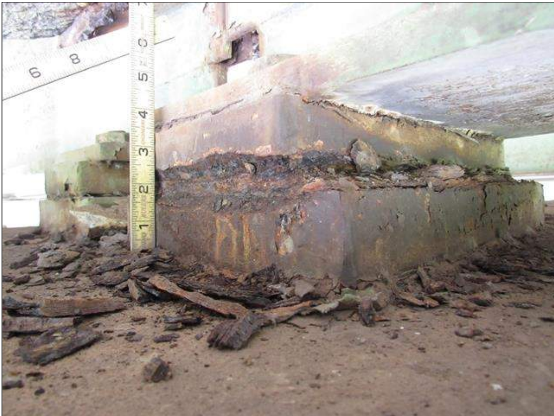
Span 2 Beam 2 - Far Bearing: PACK RUST AND HEAVY CORROSION, , SECTION LOSS HAS INITIATED
