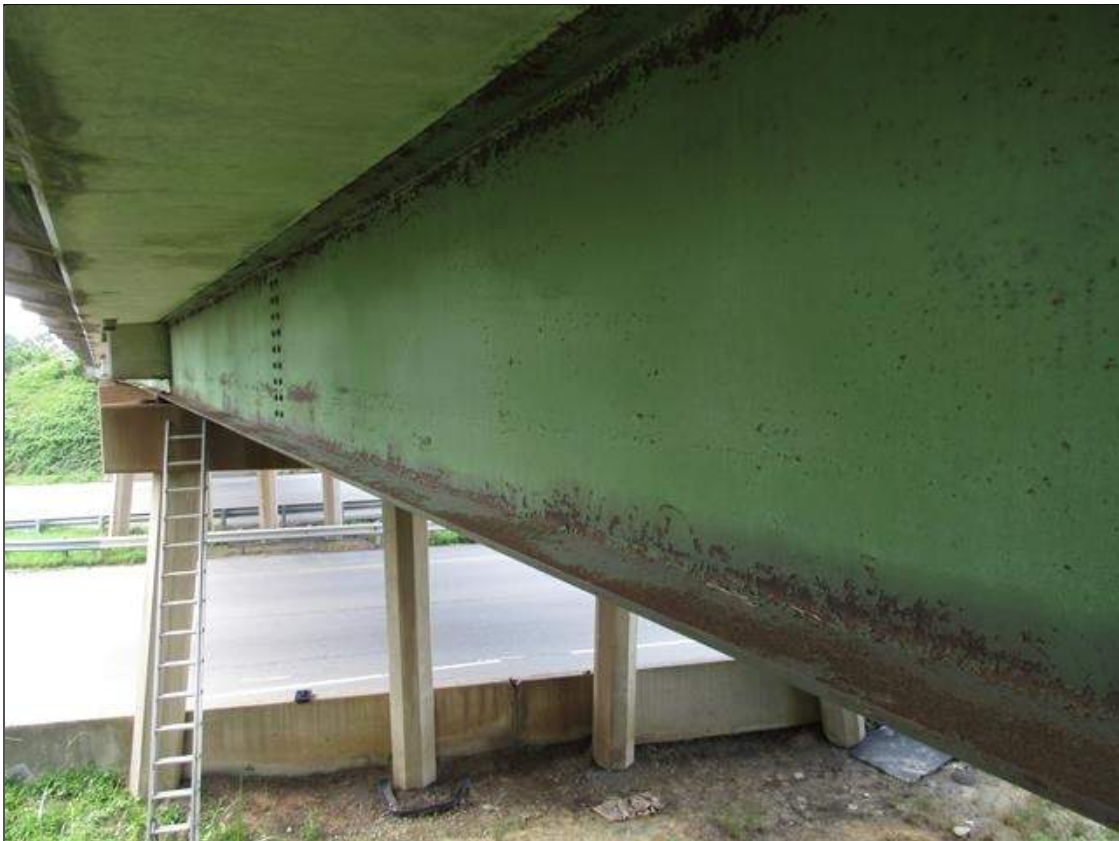
Span 4 Beam 4: MINOR SURFACE CORROSION THROUGHOUT TOP AND BOTTOM FLANGE, INTERMITTENT TO FULL LENGTH SPOTS ON WEB
