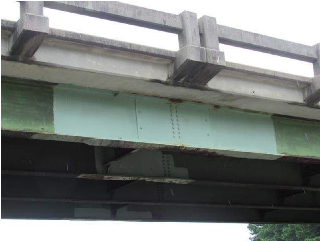
SPAN 3 BEAM 1 REPAIR
