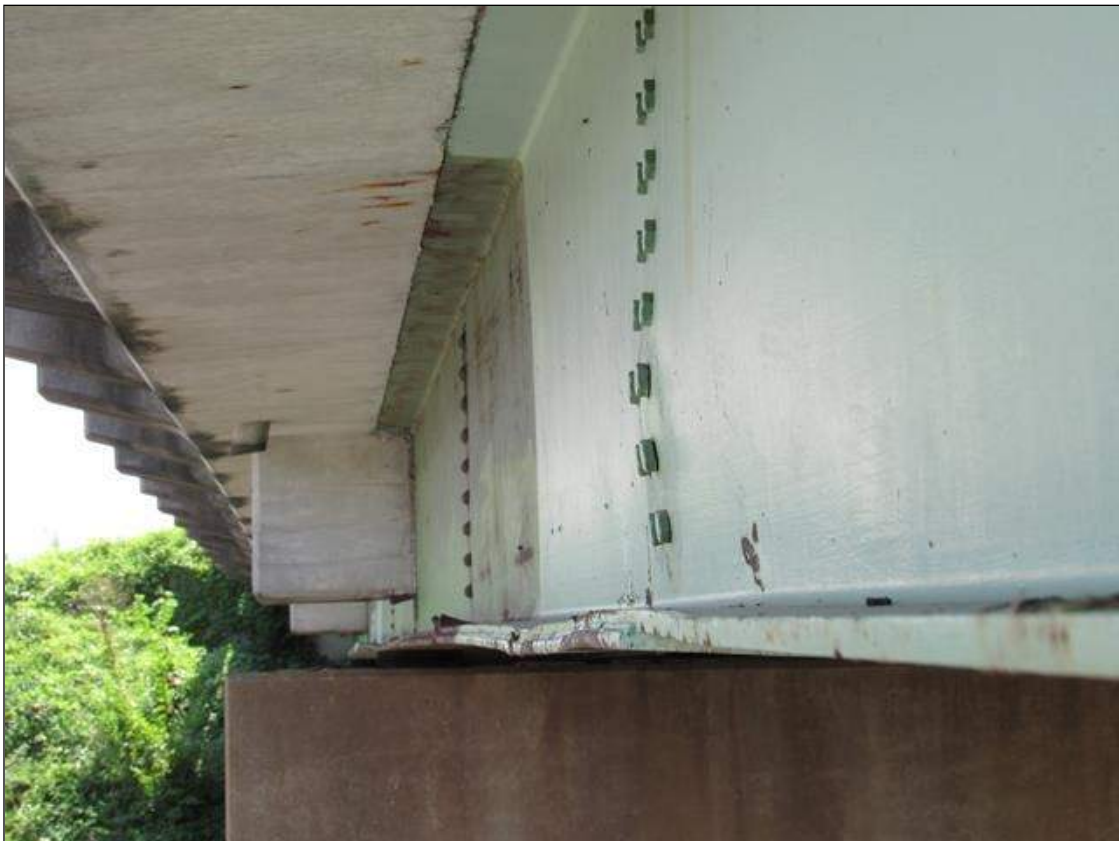
Span 2 Beam 1: BEAM 1 IN SPAN 2 IS BOWED UPWARDS 3/16 INCH FOR A LENGTH OF 3 FEET (PAR)
