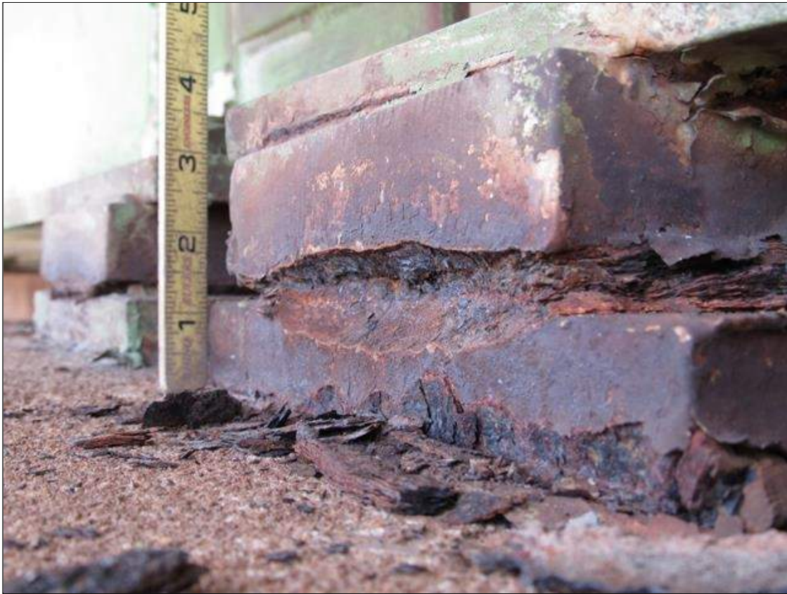
Span 2 Beam 1 - Far Bearing: PACK RUST AND HEAVY CORROSION WITH SECTION LOSS ON RIGHT AND LEFT SIDES, UP TO 5 INCH LONG X 1/4 INCH WIDE X 1/4 INCH HIGH WITH AVERAGE 3/4 INCH THICKNESS REMAINING ON MASONRY PLATE
