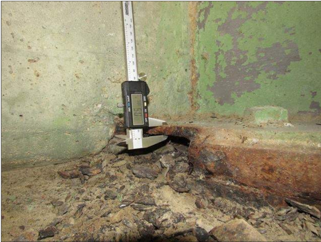
Span 1 Beam 1: 7 INCH LONG X 4 INCH WIDE AREA OF CORROSION WITH 1/8 INCH SECTION LOSS ON RIGHT BOTTOM FLANGE AT NEAR END, 1/2 INCH THICKNESS REMAINING
