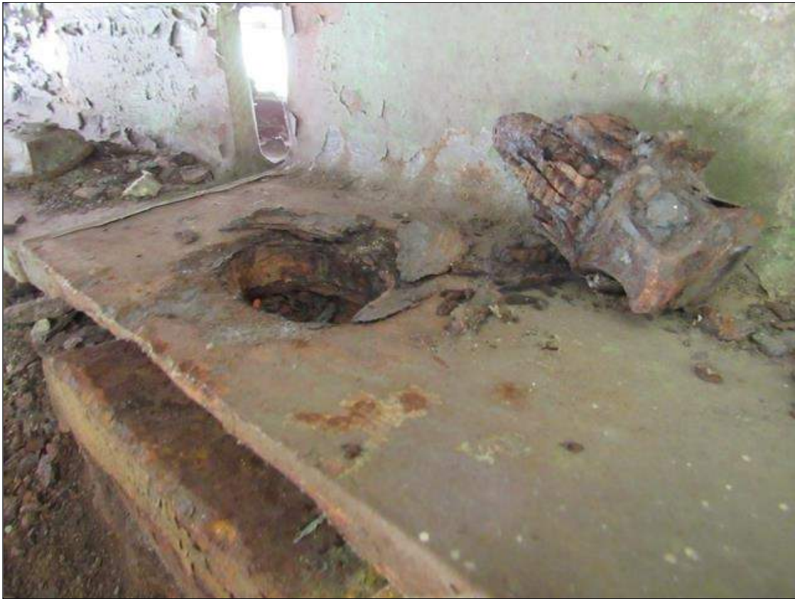
Span 4 Beam 2 - Near Bearing: MINOR CORROSION TO BEARING. RIGHT ANCHOR BOLT FULLY CORRODED (PAR)
