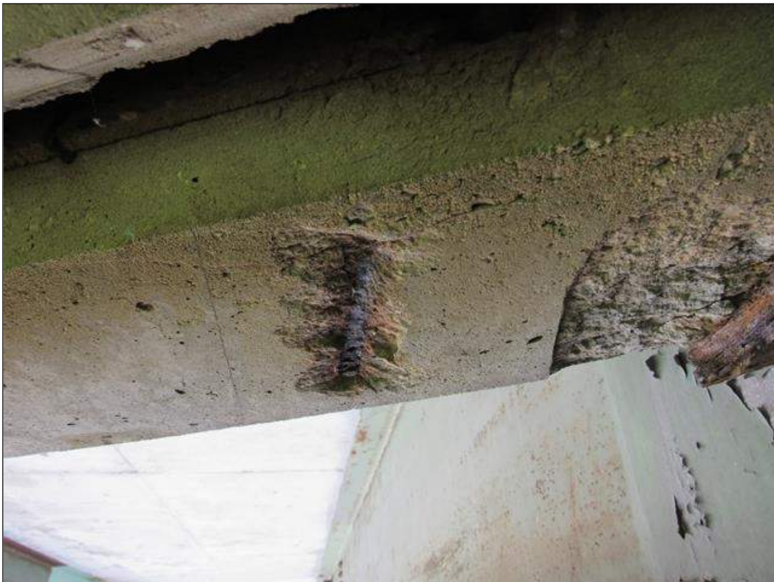
Span 3 beam 3 - 7 INCH LONG X 3 INCH WIDE X 1 DEEP SPALL WITH EXPOSED REBAR ON UNDERSIDE OF DIAPHRAGM IN BAY 3 AT BENT 3, 1 FOOT 6 INCHES FROM BEAM 3
