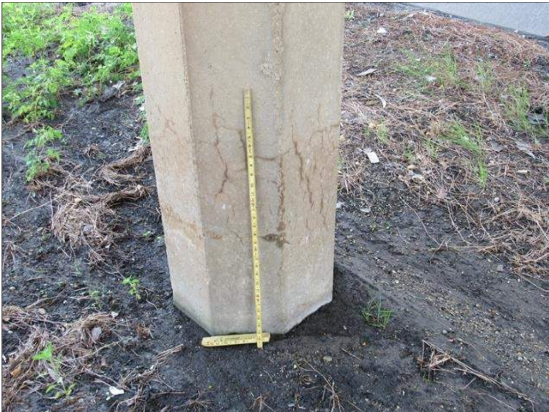
Bent 2 Pile 2: FULL PERIMETER HAIRLINE MAP CRACKING UP TO 3 FOOT HIGH AT BASE OF PILE
