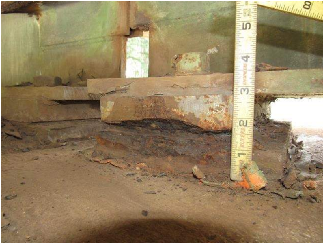
Span 2 Beam 4 - Far Bearing: HEAVY CORROSION AND PACK RUST BETWEEN PLATES, SECTION LOSS HAS INITIATED
