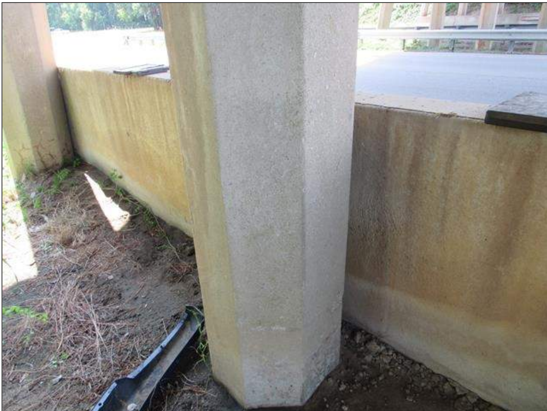
Bent 3 Pile 3: FULL PERIMETER 1/64 INCH MAP CRACKING (2 FOOT HEIGHT), BASE OF PILE - NOT OBSERVED AS OF 8/18/2022 [DID NOT OBSERVE 2024 INSPECTION]
