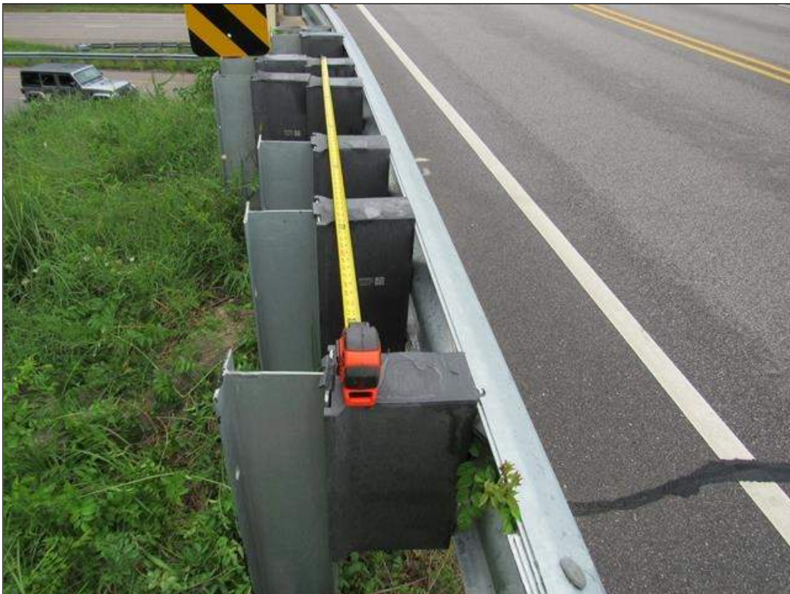
TYPICAL GUARDRAIL POST SPACING AT BRIDGE 1.55 FEET (SOUTHEAST SHOWN, ALL OTHERS SIMILAR)
