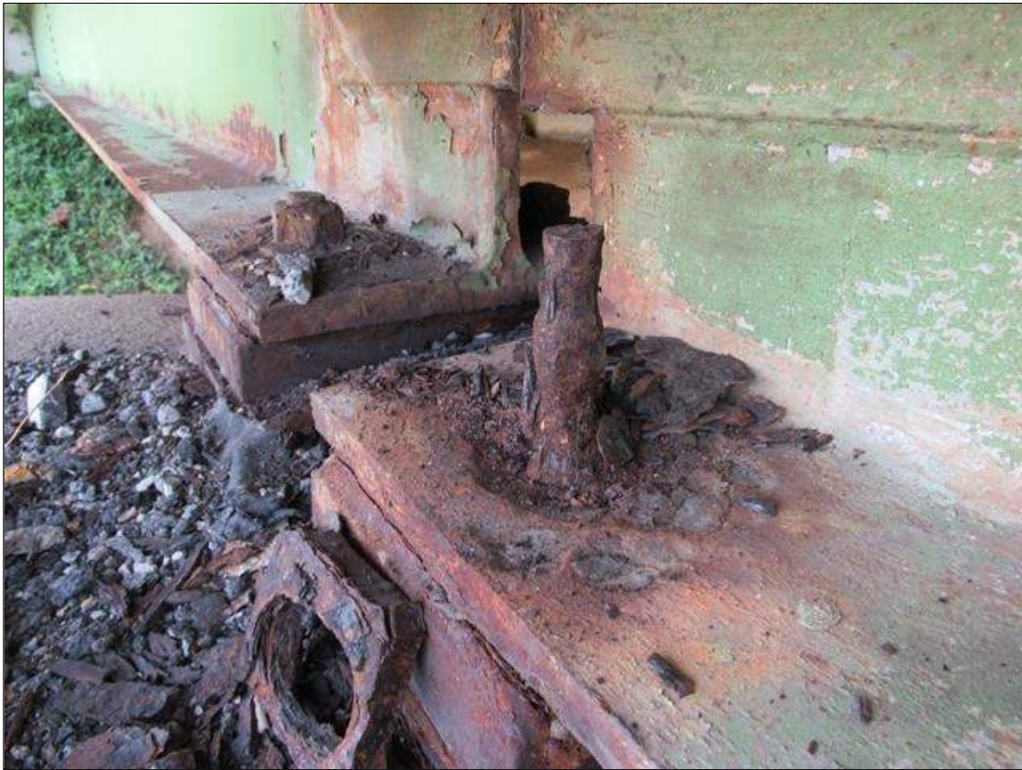
Span 3 Beam 1 - Far Bearing: PACK RUST WITH HEAVY CORROSION, CORROSION WITH 100% SECTION LOSS ON ANCHOR BOLT NUTS. SECTION LOSS HAS INITIATED ON ANCHOR BOLTS (PAR)
