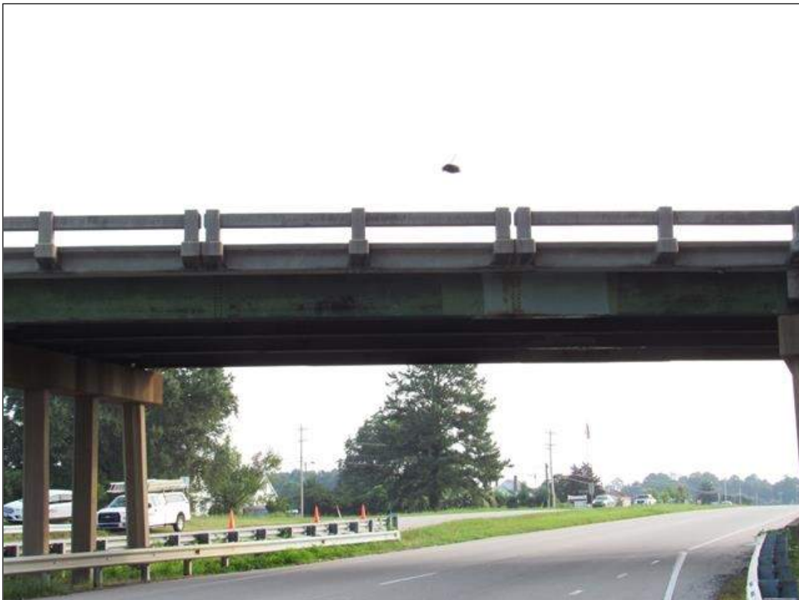
MISSING VERTICAL CLEARANCE SIGN ON BEAM 4 OVER SPAN 3.
