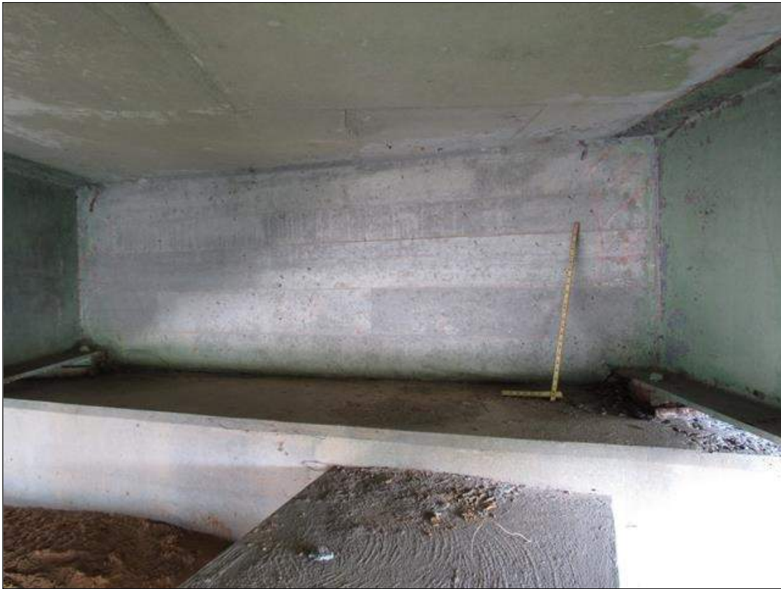
End Bent 1 Abutment: UP TO 20 INCH HIGH X 6 INCH WIDE AREA OF DELAMINATION, TOP RIGHT CORNER AT ALL BEAMS, SIMILAR AREAS OF DELAMINATION LEFT SIDE OF BEAMS 2 AND 3
