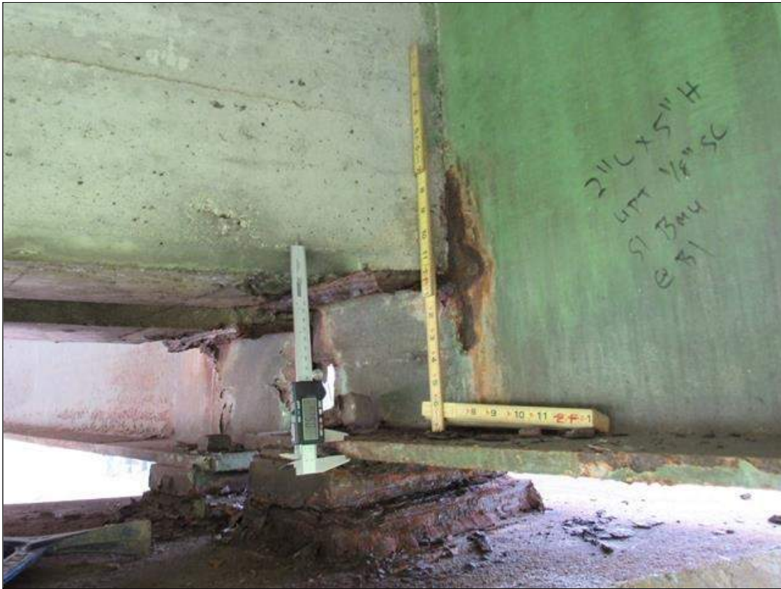
Span 1 Beam 4: 2 INCH LONG X FULL WIDTH AREA OF CORROSION WITH 1/8 INCH SECTION LOSS ON LEFT BOTTOM FLANGE AT FAR BEARING (1/2 INCH THICKNESS REMAINING) AND 1/16 INCH SECTION LOSS IN WEB AT DIAPHRAGM 2 INCH WIDE X 6 INCH HIGH (9/16 INCH REMAINING)
