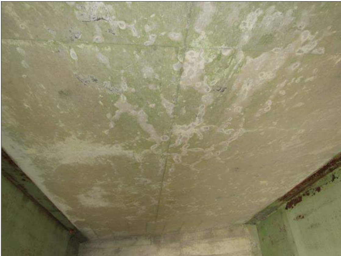
Span 1 Deck: HAIRLINE MAP CRACKING ALONG UNDERSIDE IN ALL BAYS AND OVERHANGS
