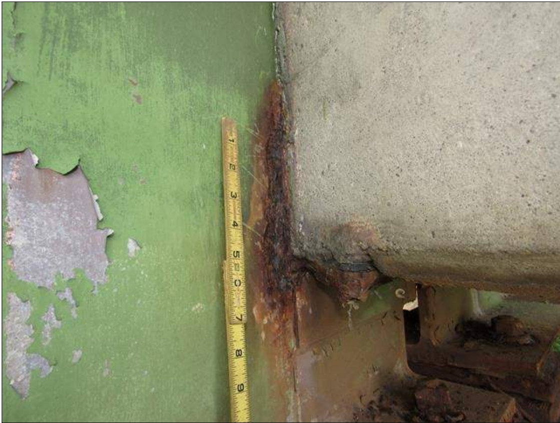
Span 3 Beam 4: ACTIVE CORROSION IN WEB AT FAR END DIAPHRAGM, 8 INCHES HIGH X 1.5 INCHES WIDE WITH 1/16 INCH SECTION LOSS (9/16 INCH REMAINING)
