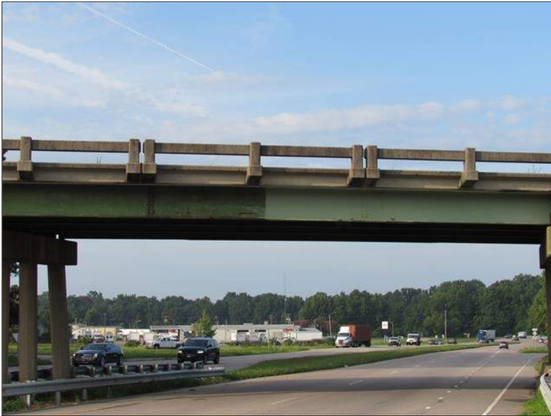
MISSING VERTICAL CLEARANCE SIGN ON BEAM 1 OVER SPAN 2.
