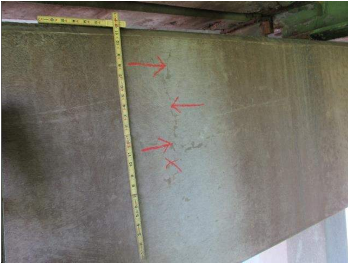
Bent 1 Cap 1: 1/32 INCH VERTICAL CRACKING ON BOTH FACES
