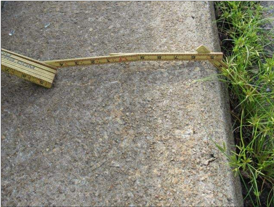
Span 1 Left Bridge Rail: HAIRLINE WRAP AROUND CRACKS IN CURB
