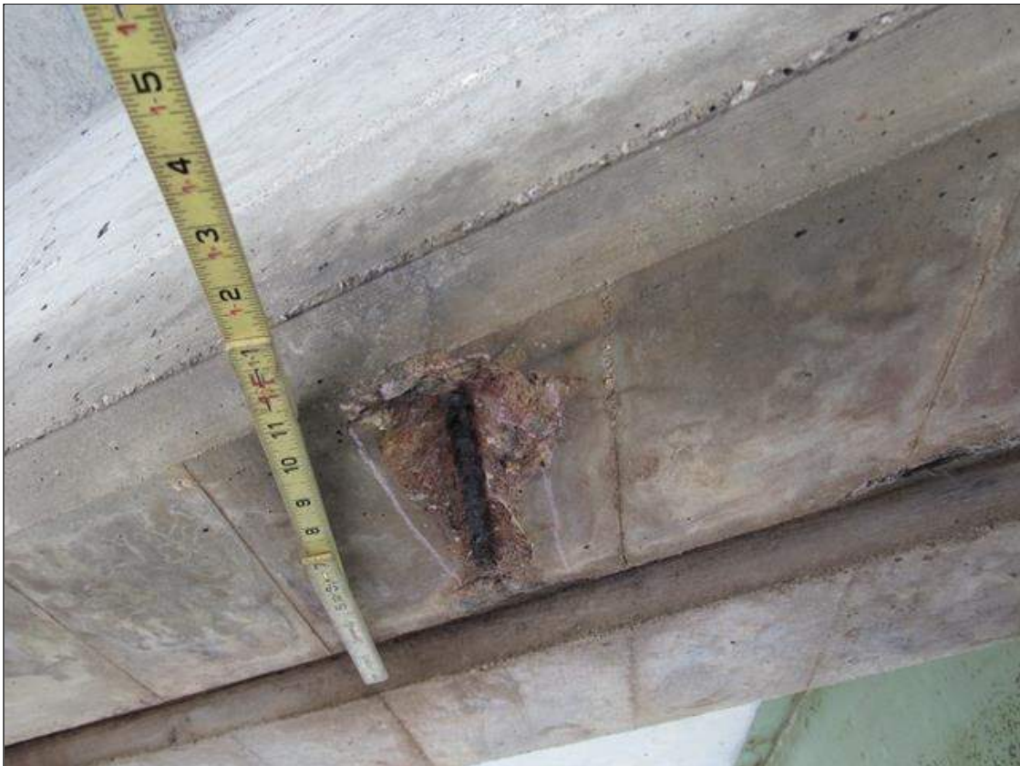
Span 3 Beam 2 - 7 INCH LONG X 3 INCH WIDE X 1 DEEP SPALL WITH EXPOSED REBAR ON UNDERSIDE OF DIAPHRAGM IN BAY 2 AT BENT 2, 2 FEET 6 INCHES FROM BEAM 2
