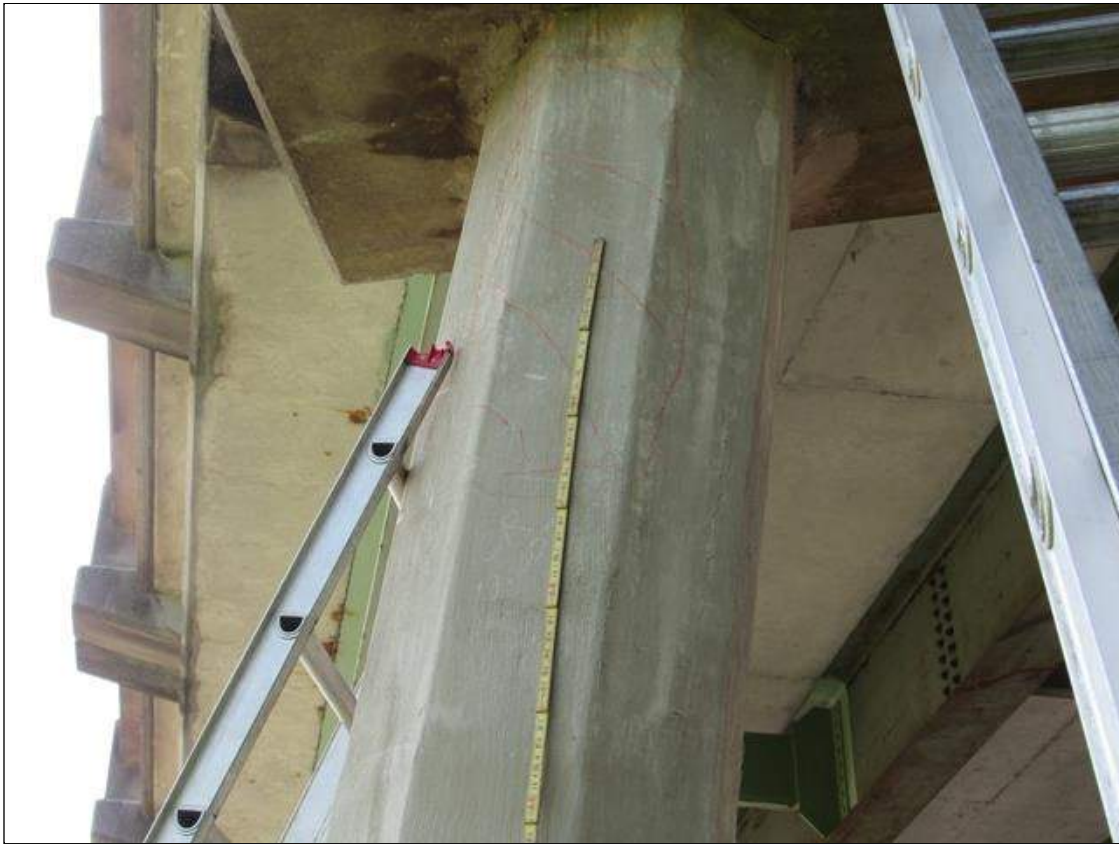
Bent 1 Pile 1: 12 INCH X 8 INCH X 5 INCH DEEP SPALL WITH EXPOSED REBAR ON WEST FACE AT TOP - DEFECT IS AN UNSOUND PATCH WITH A 13 INCHES WIDE X 3 FOOT HIGH AREA OF DELAMINATION ON WEST FACE, 1 FOOT BELOW CAP AS 8/18/2022 (PAR)
