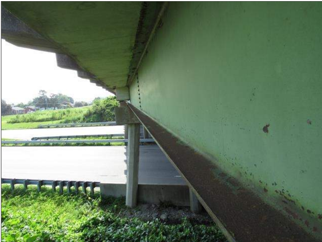
Span 1 Beam 1: MINOR SURFACE CORROSION THROUGHOUT TOP AND BOTTOM FLANGE, INTERMITTENT TO FULL LENGTH SPOTS ON WEB
