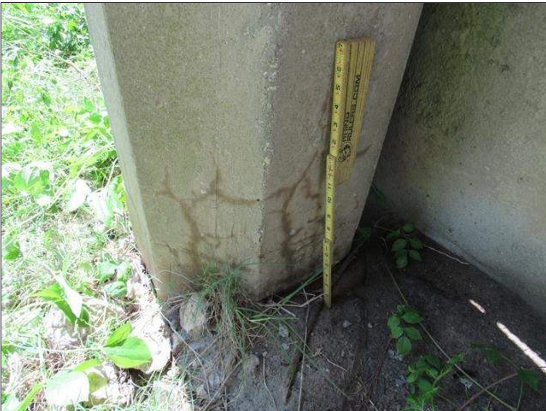
Bent 3 Pile 4: FULL PERIMETER HAIRLINE MAP CRACKING (16 INCH HIGH), BASE OF PILE
