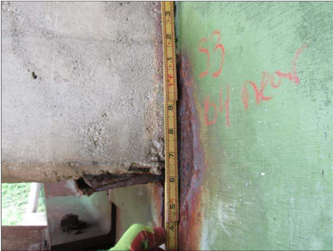
Span 3 Beam 4: ACTIVE CORROSION IN RIGHT SIDE OF WEB AT NEAR END DIAPHRAGM, 8 INCH HIGH X 2 INCH WIDE WITH 1/8 INCH SECTION LOSS (1/2 INCH REMAINING) (PAR)
