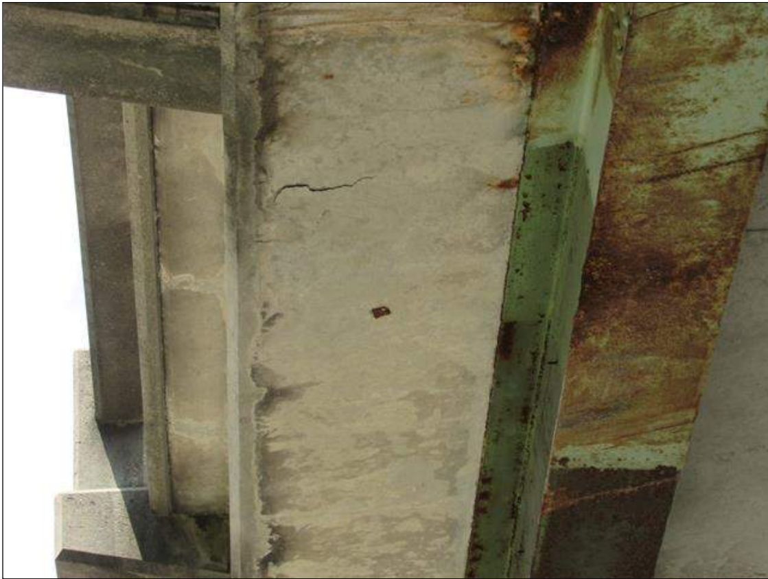
Span 3 Deck: APPROXIMATELY 1 FOOT LONG X 3 INCH WIDE AREA OF DELAMINATION IN RIGHT OVERHANG OVER CENTERLINE OF NORTHBOUND LANES - NCDOT NOTIFIED 8/13/2022 (PAR)
