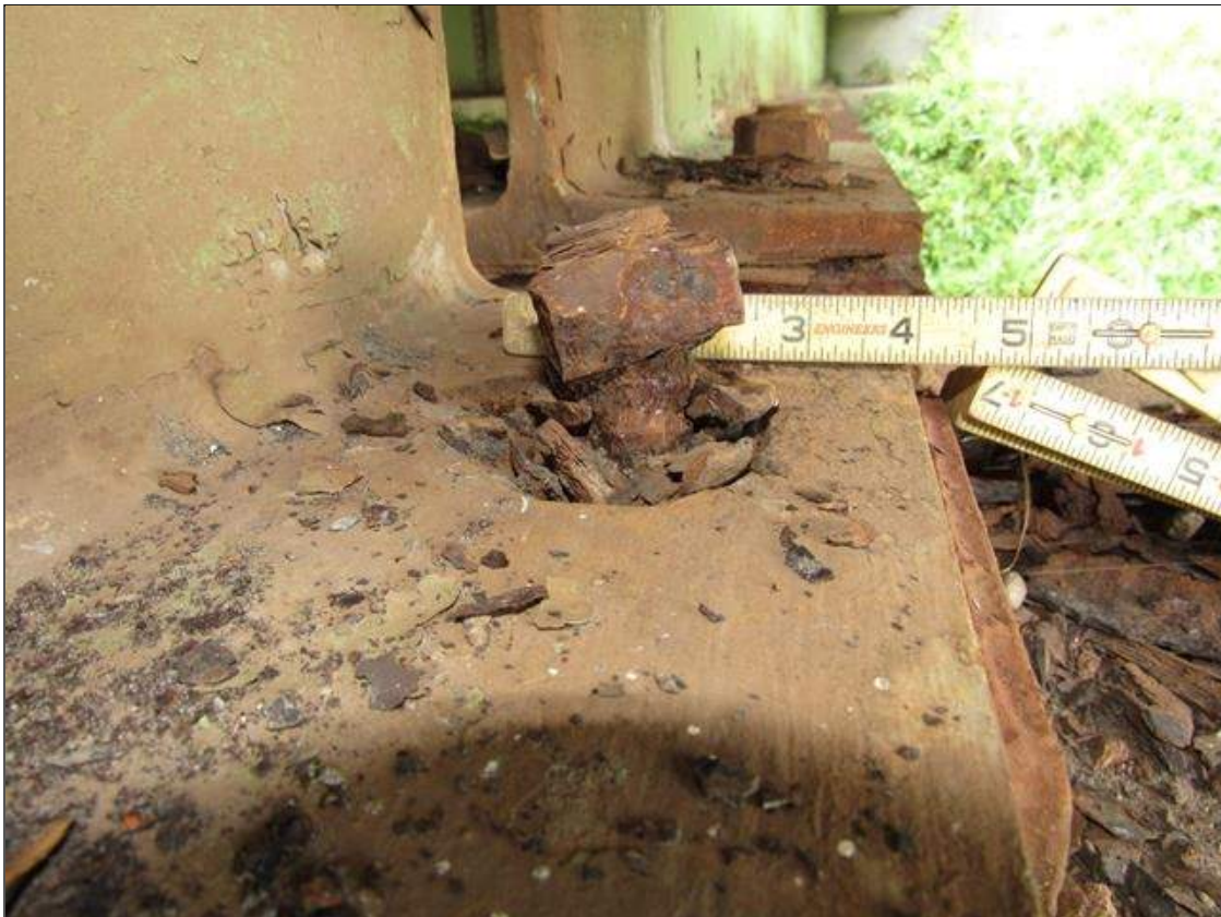
Span 3 Beam 4: BEAM 4 FAR BEARING EAST ANCHOR BOLT NUT NOT FULLY ENGAGED AND BOLT CORRODED WITH APPROXIMATELY 50% SECTION LOSS (PAR)
