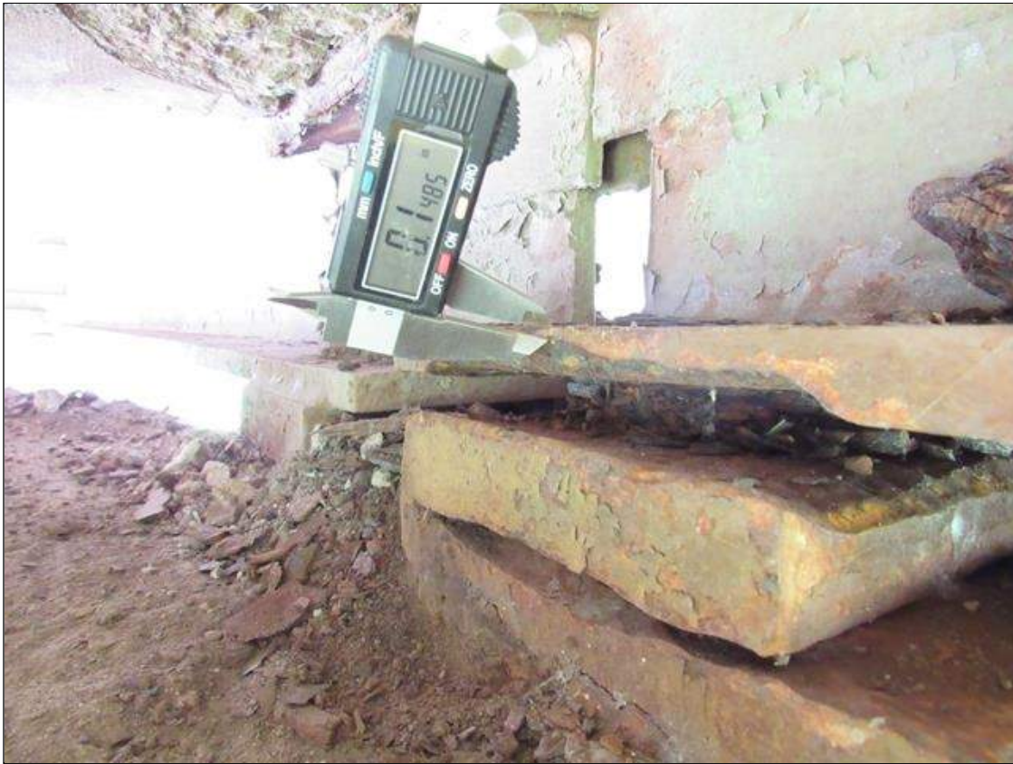
Span 4 Beam 2: 7 INCH LONG X 4 INCH WIDE OF CORROSION WITH SECTION LOSS DOWN TO 1/8 INCH THICKNESS REMAINING ON RIGHT BOTTOM FLANGE AT BENT 3, AVERAGE 7/16 INCH THICKNESS REMAINING (PAR)
