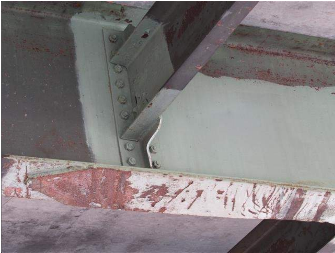
BAY 1 DIAPHRAGM GUSSET PLATE AT BEAM 2 IS DEFORMED FROM IMPACT DAMAGE
