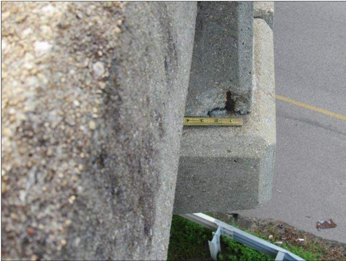
Span 2 Right Bridge Rail: RAIL POST AT FAR END, SPALL WITH EXPOSED REBAR 4 INCH HIGH X 4 INCH WIDE X 1/2 INCH DEEP AT BASE ON SOUTH FACE
