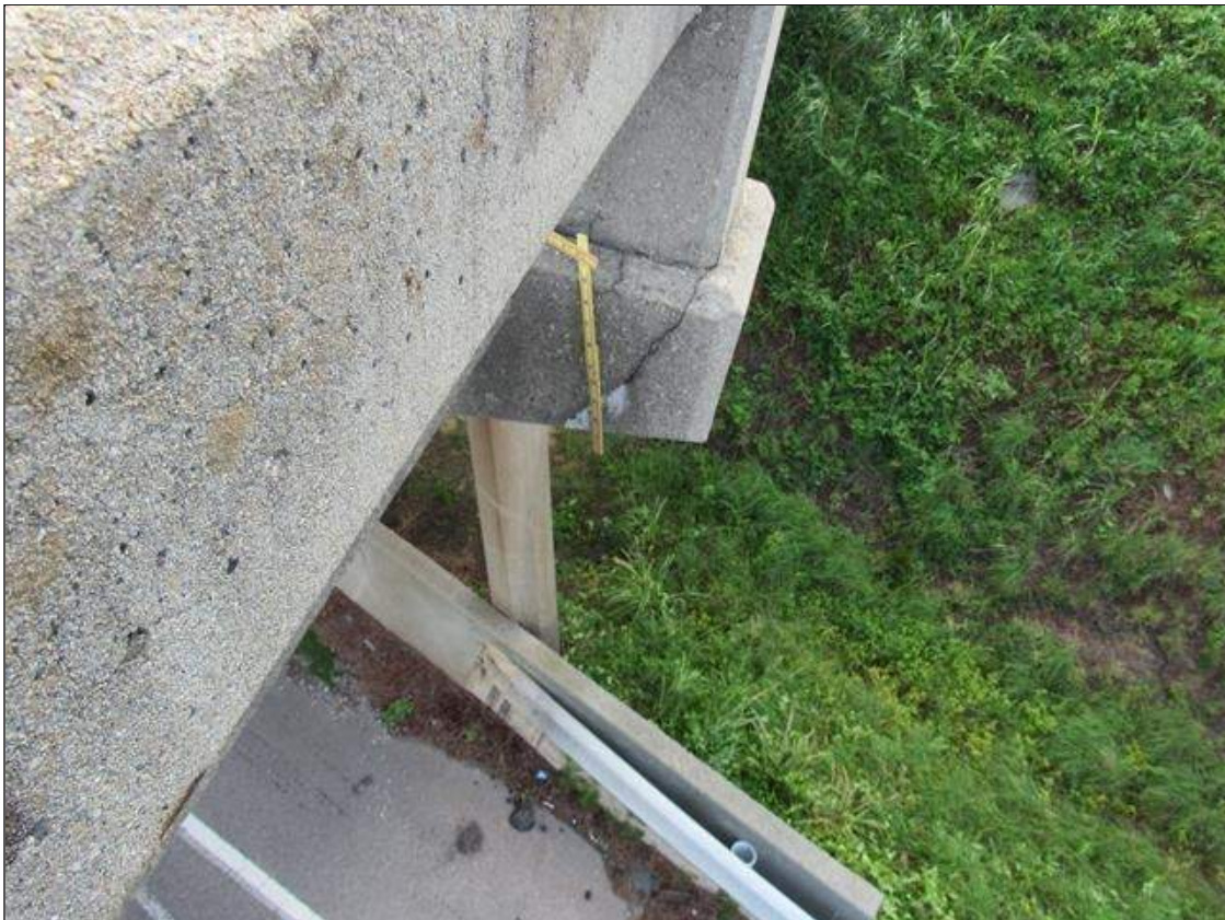
Span 3 Right Bridge Rail: 0.03 INCH WIDE DIAGONAL CRACK WITH EFFLORESCENCE ON EAST AND WEST FACE OF SUPPORT BLOCK AT POST 8
