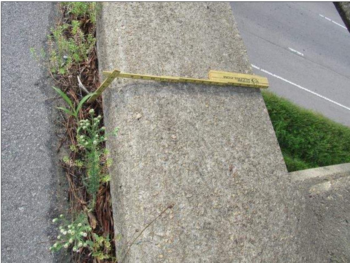
Span 1 Right Bridge Rail: HAIRLINE WRAP AROUND CRACKS IN CURB
