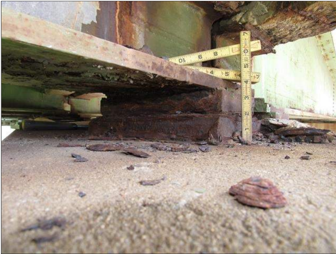
Span 1 Beam 4 - Far Bearing: MINOR SCALE AND PACK RUST, NO MEASURABLE SECTION LOSS
