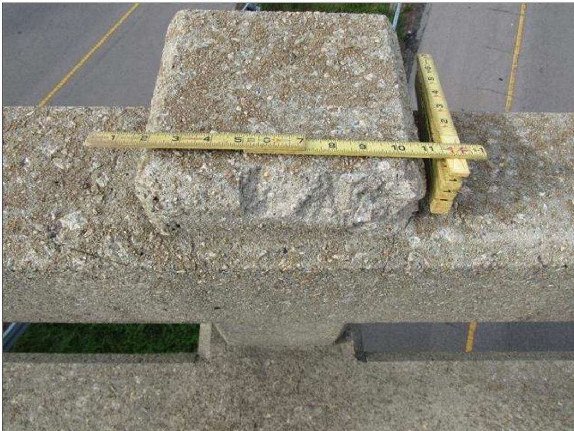
Span 2 Right Bridge Rail: 7 INCH LONG X 3 INCH HIGH X 1/2 INCH DEEP SPALL WITH EXPOSED REBAR ON SOUTHWEST CORNER OF RAIL POST AT FAR END
