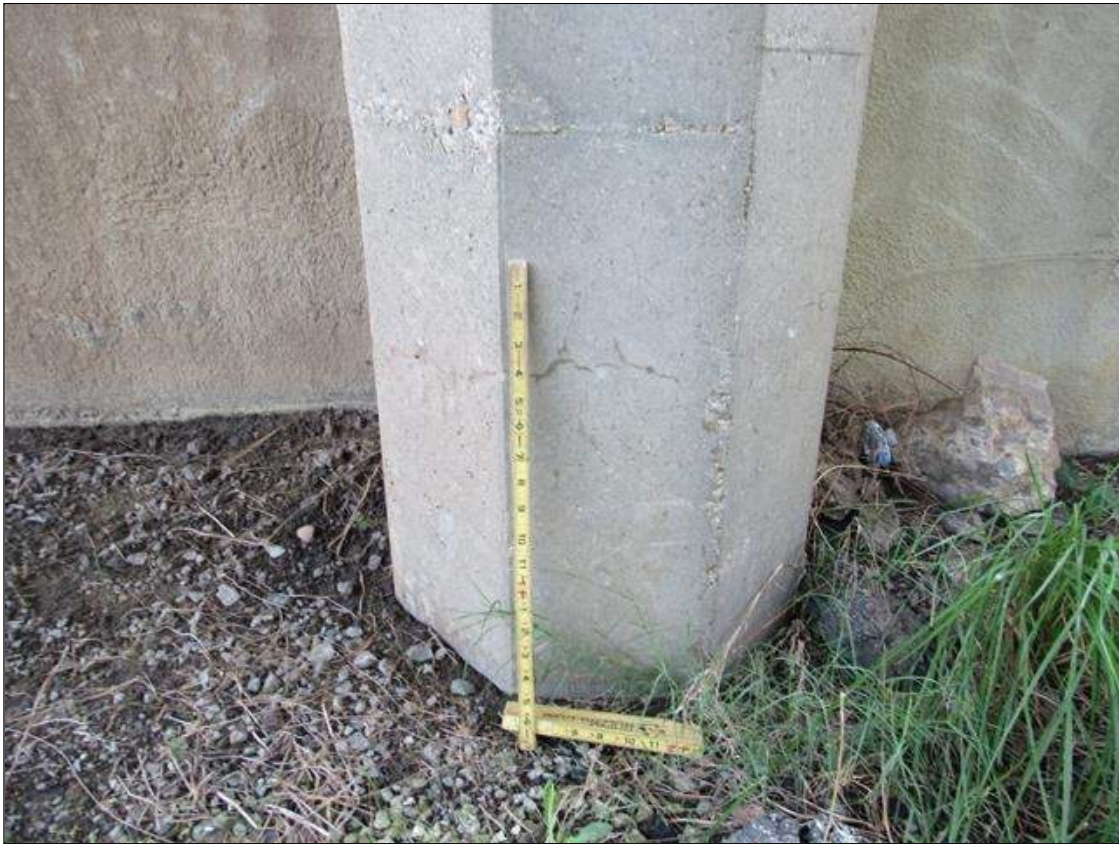
Bent 1 Pile 3: HAIRLINE MAP CRACKING AT BASE
