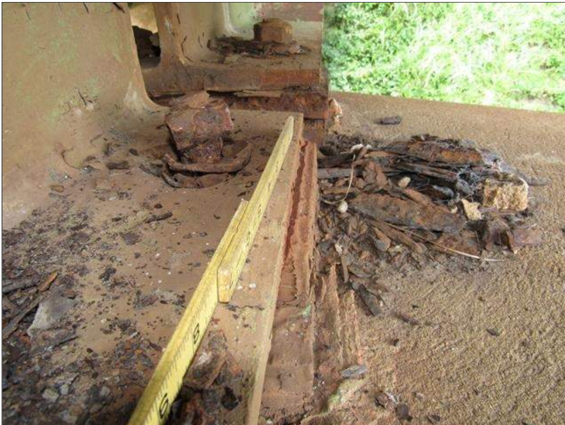
Span 3 Beam 4 - Far Bearing: PACK RUST AND HEAVY CORROSION, CRACKED WELD ON RIGHT SIDE OF BEARING AND MASONRY PLATE
