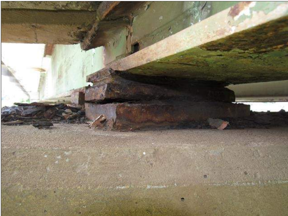
Span 4 Beam 4 - Near Bearing: PACK RUST AND HEAVY CORROSION
