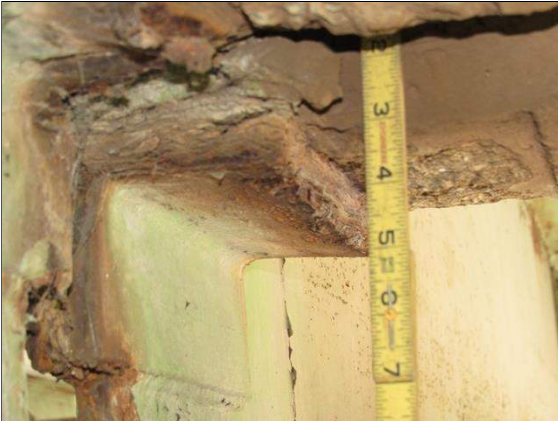
END DIAPHRAGM STEEL SUPPORT ANGLES OVER BENT 1 WITH PACK RUST UP TO 1 INCH (SPAN 2 BAY 3 AT BEAM 3 SHOWN)
