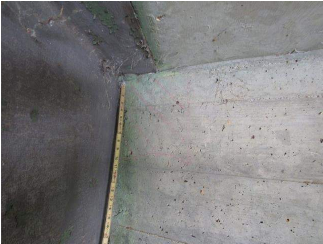
End Bent 2 Abutment: 1 FOOT LONG X 11 INCH HIGH AREA OF DELAMINATION ADJACENT RIGHT TOP FLANGE OF BEAM 2
