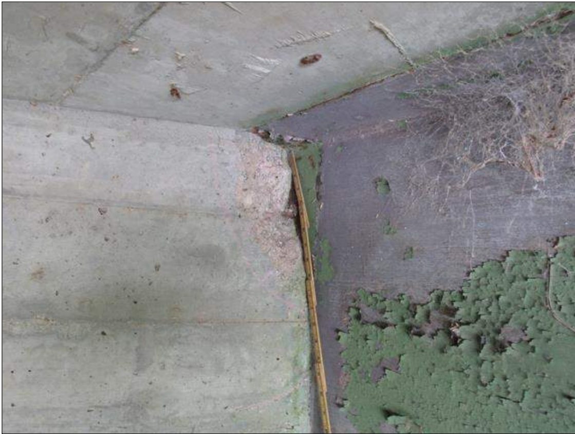
End Bent 2 Abutment: SPALL WITH EXPOSED REBAR (1 FOOT HIGH X 6 INCH WIDE X 3 INCH DEEP) TOP CORNER LEFT OF BEAM 2
