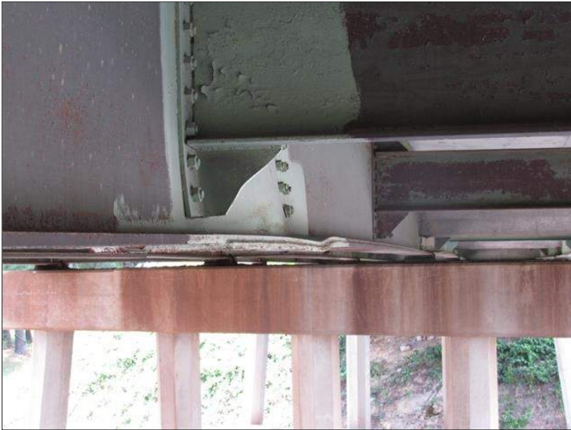
Span 3 Beam 2: 3 FOOT LONG AREA OF MODERATE IMPACT DAMAGE LOCATED 18 FEET FROM EAST END, BOTTOM FLANGE IS BOWED UPWARDS 1 1/4 INCH FOR A LENGTH OF 3 FEET, 1 3/4 INCH LONG X 1/4 INCH DEEP GOUGE IN BOTTOM FLANGE COVER PLATE, AND BEAM IS BOWED TOWARDS THE NORTH 1 3/4 INCH (PAR)
