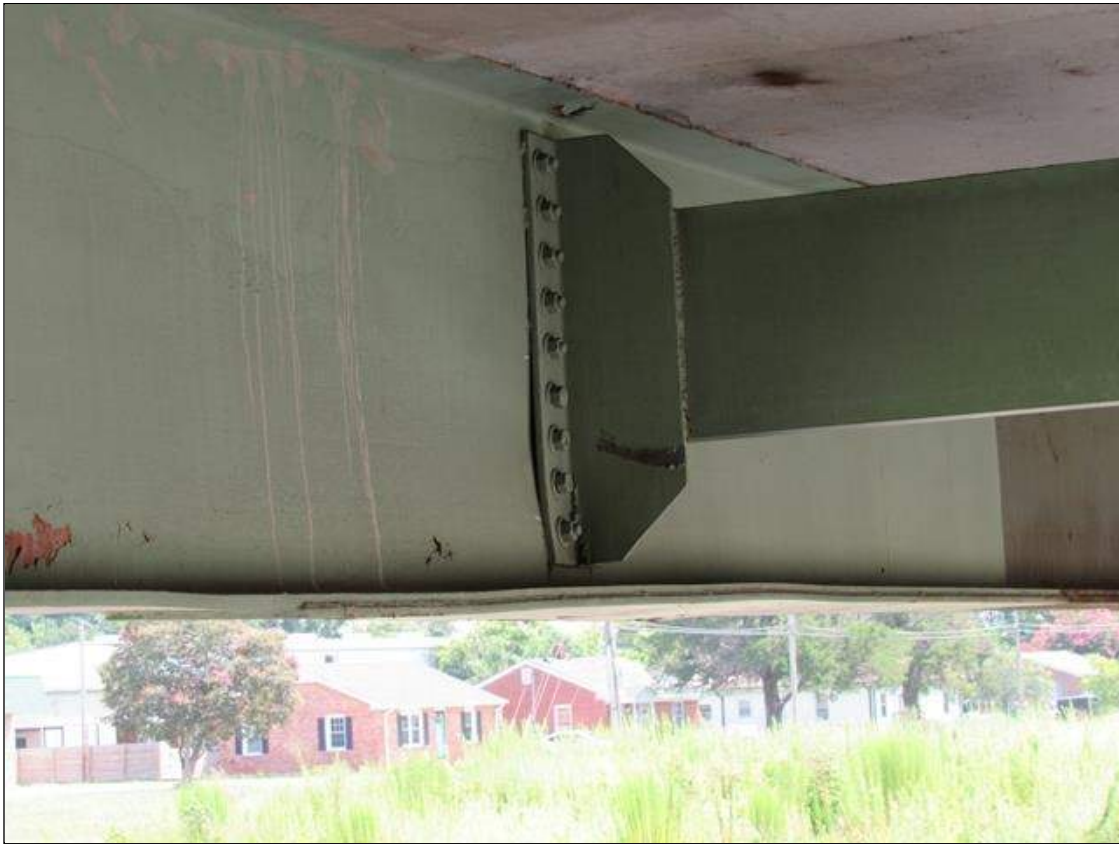
Span 2 Beam 1: BEAM 1 IN SPAN 2 WEB IS BOWED AWAY FROM INTERMEDIATE DIAPHRAGM 1 IN BAY 1 FOR 1/2 INCH FOR A LENGTH OF 10 INCH (PAR ISSUED)
