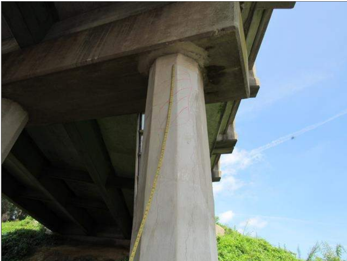
Bent 1 Pile 1: EAST FACE AT 1 FOOT BELOW CAP UNSOUND PATCH 2 FEET HIGH UP TO 14 WIDE
