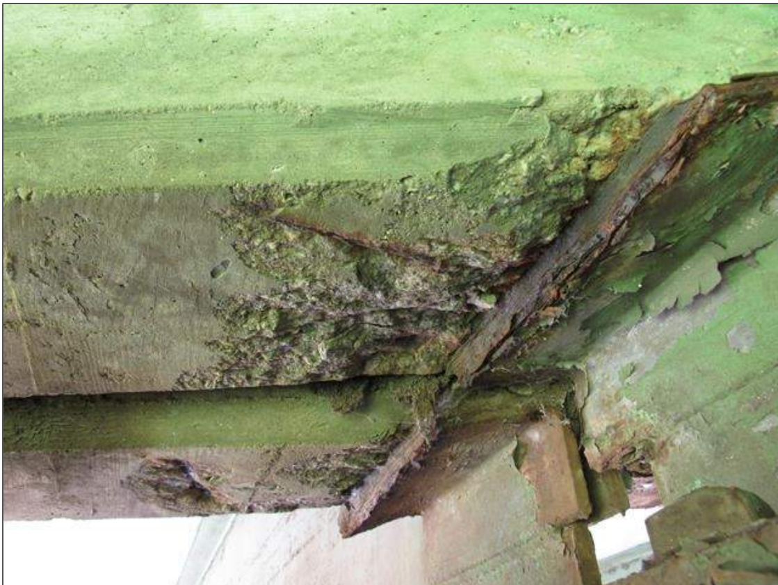
MULTIPLE END DIAPHRAGMS OVER BENTS WITH SPALLS, SOME WITH EXPOSED REBAR, ADJACENT TO BEAMS [TYPICAL 8 INCHES LONG X 7 INCHES WIDE X 1 INCH DEEP] (SPAN 1 BAY 2 SHOWN)
