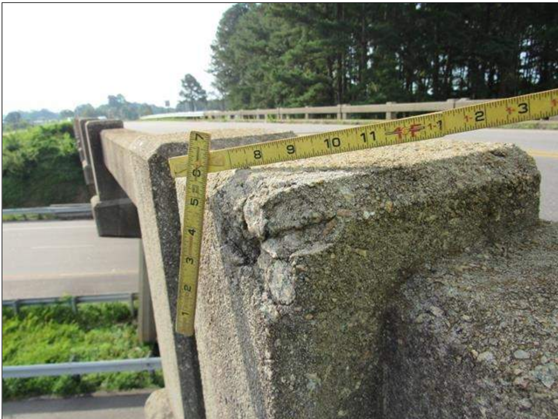
Span 2 Left Bridge Rail: 3 INCH LONG X 4 INCH WIDE X 2 INCH DEEP SPALL AND DELAMINATION ON TOP EXTERIOR CORNER OF THIRD RAIL POST FROM BENT 1
