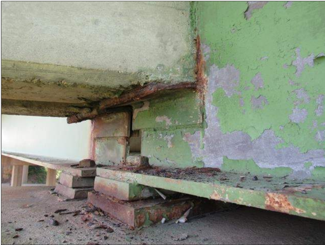
Span 1 Beam 1: 2 INCH LONG X 5 INCH HIGH AREA OF CORROSION WITH SECTION LOSS ON LEFT FACE OF WEB ADJACENT TO DIAPHRAGM AT BENT 1, 1/2 INCH THICKNESS REMAINING [NO SECTION LOSS OBSERVED 2024 INSPECTION]
