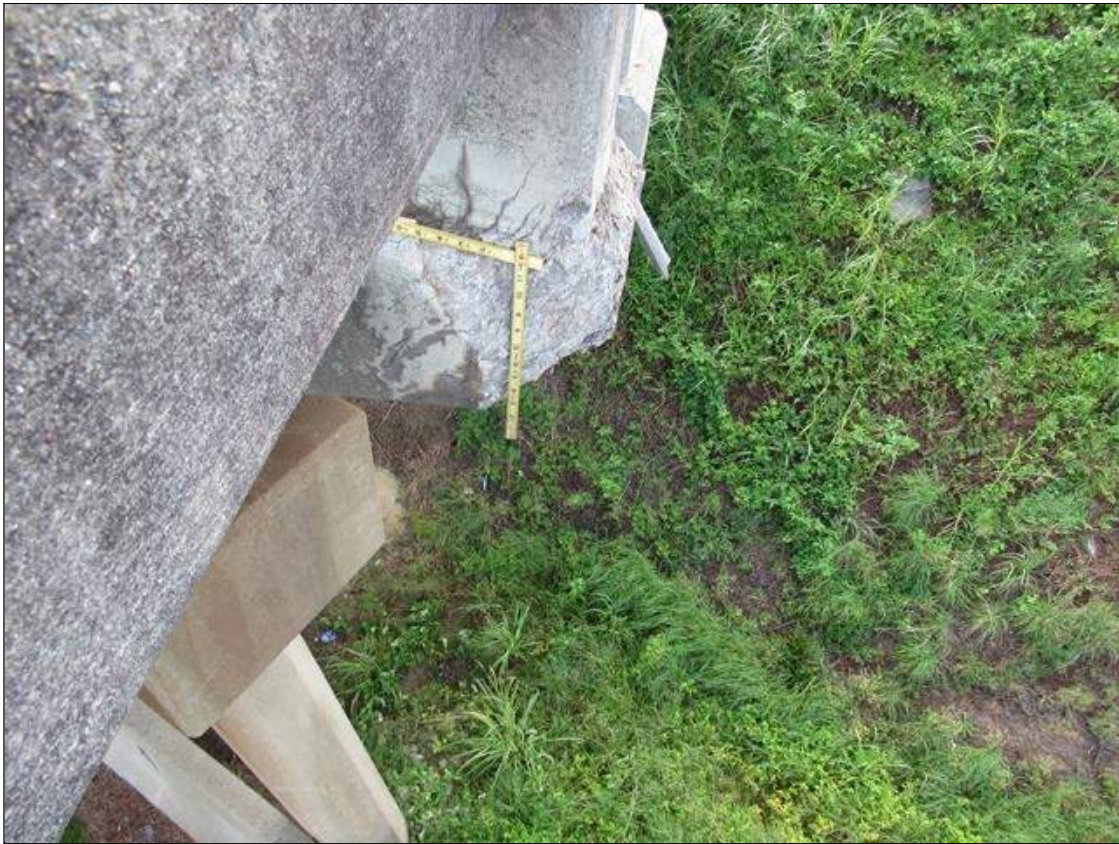
Span 3 Right Bridge Rail: SPALL 11 INCH HIGH X 8 INCH WIDE X 4 INCH DEEP, NO EXPOSED REBAR BOTTOM OF RAIL POST, FAR END (PAR)
