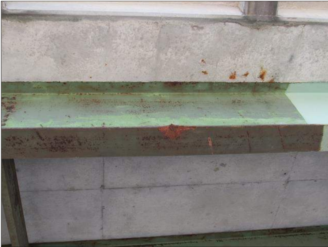
Span 2 Beam 1: MINOR IMPACT DAMAGE ON LEFT BOTTOM FLANGE OVER LEFT LANE
