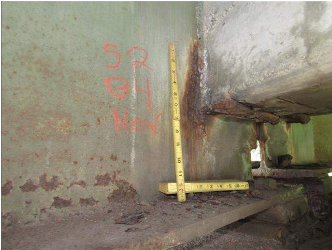
Span 2 Beam 4: ACTIVE CORROSION IN WEB AT NEAR END DIAPHRAGM WITH 1/16 INCH SECTION LOSS, 2 INCHES WIDE X 8 INCHES HIGH (9/16 INCH REMAINING)
