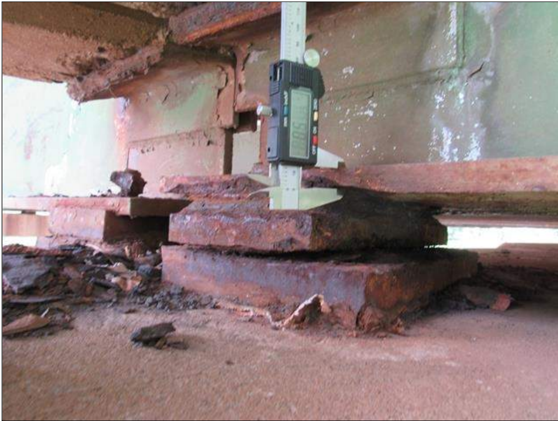
Span 4 Beam 4: 2 INCH LONG X FULL WIDTH AREA OF CORROSION WITH SECTION LOSS ON UNDERSIDE OF BOTTOM RIGHT FLANGE AT NEAR BEARING, 1/2 INCH THICKNESS REMAINING
