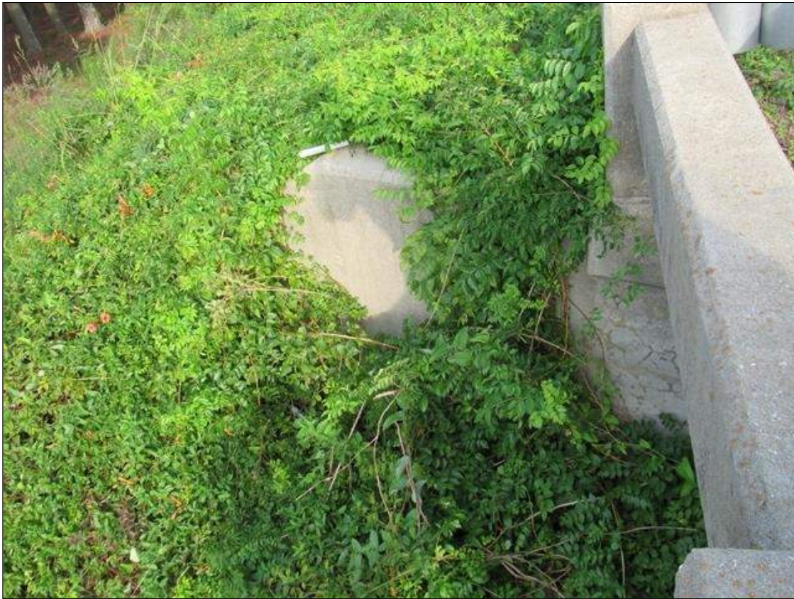
VEGETATION GROWTH ENCROACHING WINGWALLS AT ALL CORNERS
