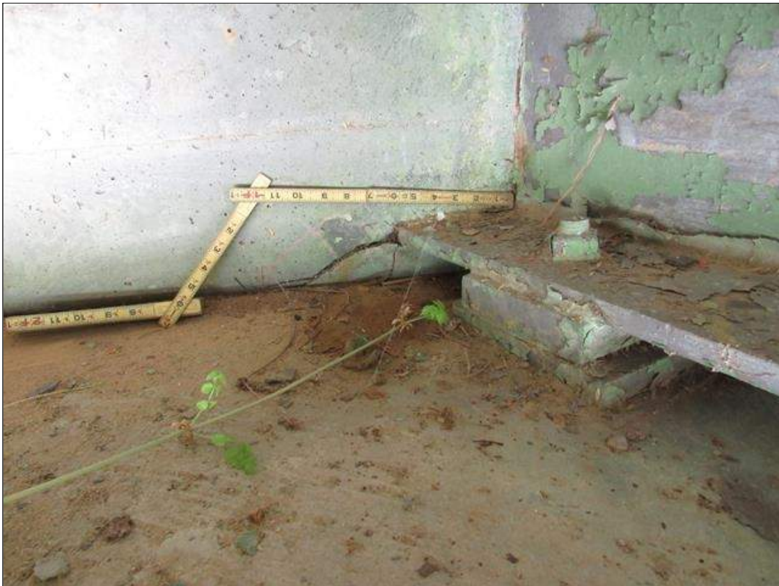
End Bent 2 Abutment: 1 FOOT LONG X 4 INCH HIGH AREA OF DELAMINATION WITH 1/4 INCH WIDE CRACKING, ADJACENT TO LEFT BOTTOM FLANGE OF BEAM 2
