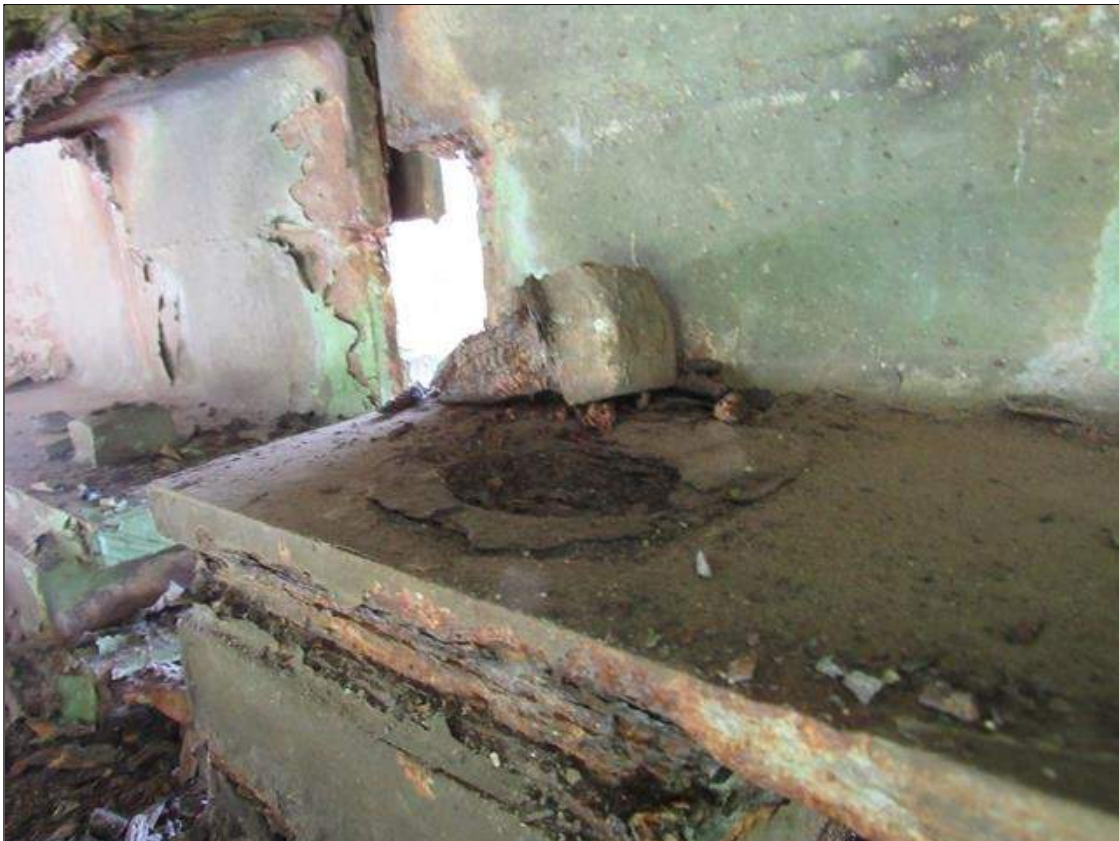
Span 1 Beam 4 - Far Bearing: LEFT ANCHOR BOLT IS BROKEN (PAR)
