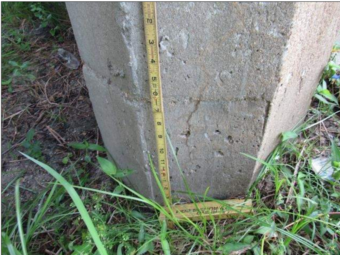
Bent 1 Pile 4: HAIRLINE VERTICAL CRACKING AT BASE
