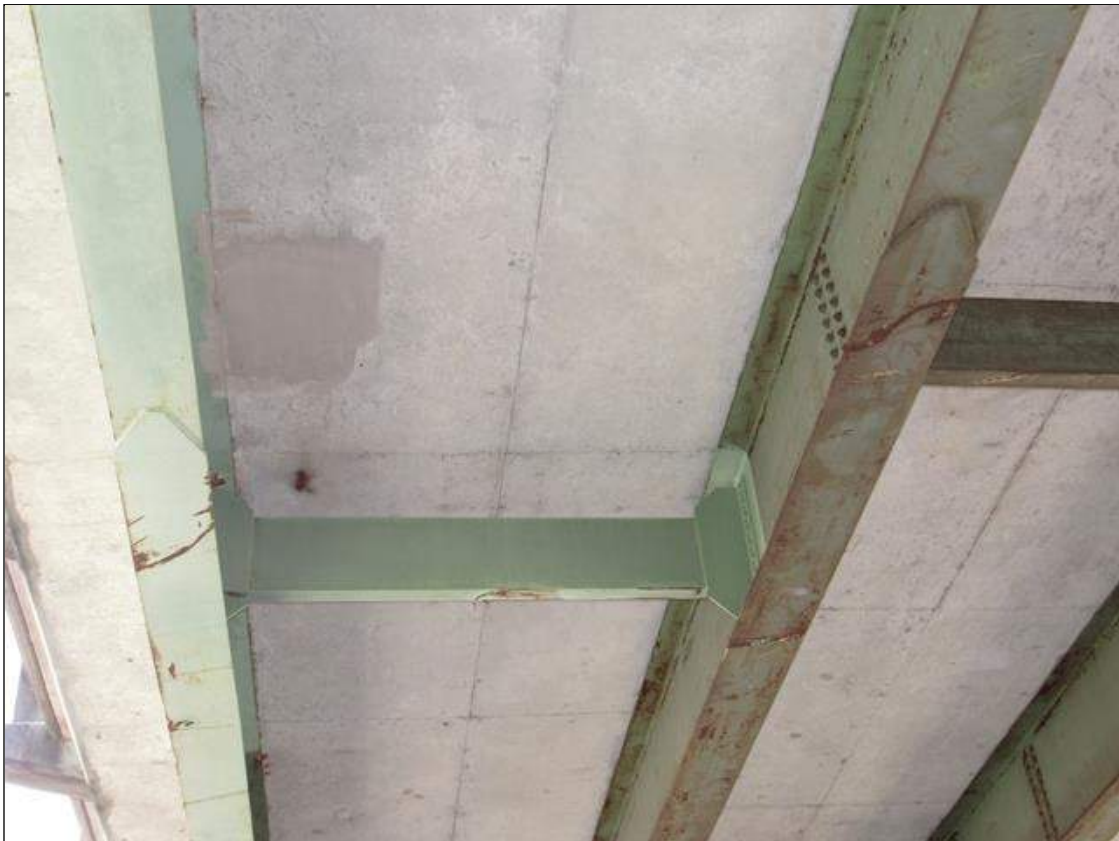
Span 2 Beam 2: BOTTOM FLANGE, MINOR SCRAPES TO BOTTOM FACE OVER RIGHT TRAVEL LANE
