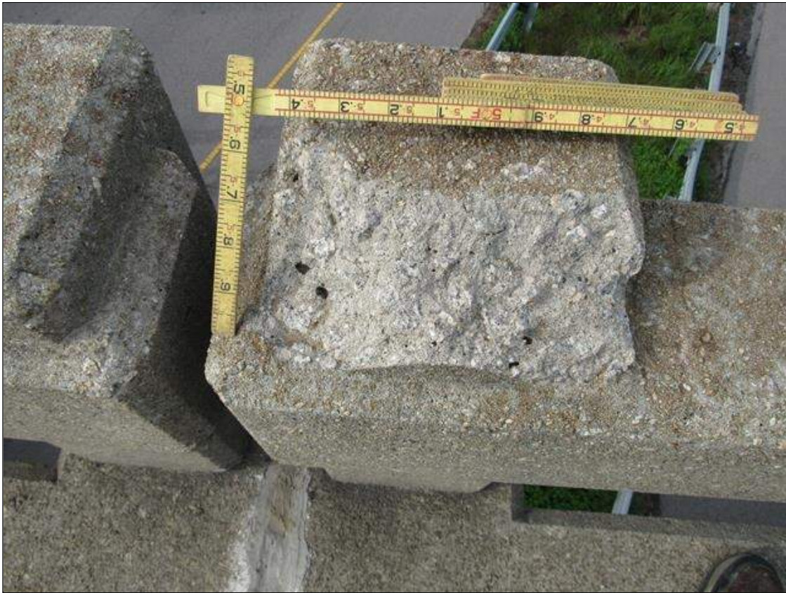
Span 2 Right Bridge Rail: SPALL 8 INCH LONG X 4 INCH WIDE X 2 INCH DEEP, TOP OF RAIL POST AT FAR END
