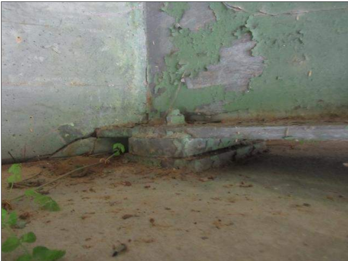
SIMILAR BEARING AT END BENTS (END BENT 2 AT BEAM 2 SHOWN)
