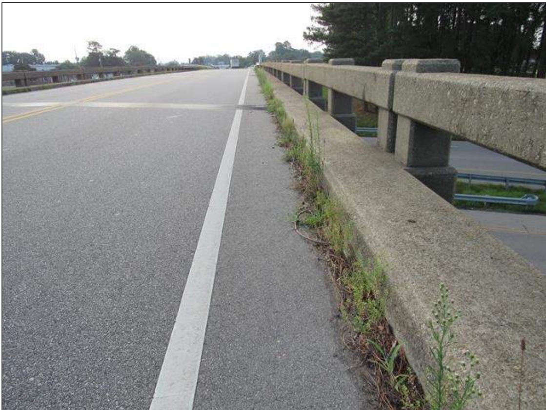
UP TO 6 INCH WIDE AREAS OF DIRT AND DEBRIS ACCUMULATION WITH VEGETATION GROWTH ALONG BRIDGE RAILS.
