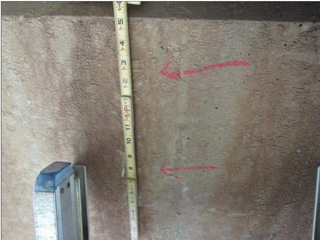
Bent 3 Cap 1: HAIRLINE VERTICAL CRACKING ON BOTH FACES
