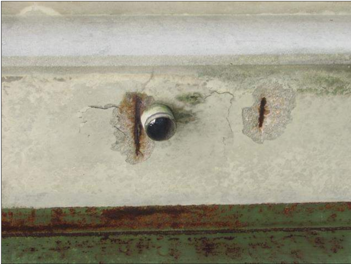
Span 3 Deck: TWO SPALLS WITH EXPOSED REBAR APPROXIMATELY 1 FOOT LONG X 5 INCH WIDE X 1/2 INCH DEEP WITH ADJACENT AREA OF DELAMINATION IN UNDERSIDE OF RIGHT OVERHANG, LOCATED AT DRAIN OVER RIGHT SHOULDER OF NORTHBOUND LANES (PAR)
