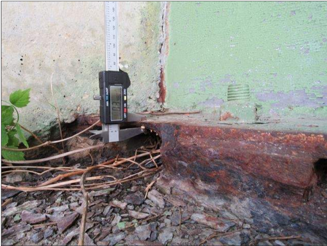
Span 4 Beam 1: 4 INCH LONG X FULL WIDTH CORROSION WITH SECTION LOSS ON LEFT BOTTOM FLANGE AT FAR END, 5/16 INCH THICKNESS REMAINING (PAR)
