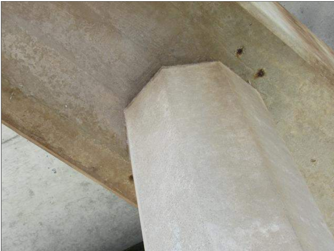
Bent 2 Cap 1: SCATTERED SPALLS WITH EXPOSED REBAR UP TO 1 INCH DIAMETER X 1/2 INCH DEEP IN UNDERSIDE OF CAP
