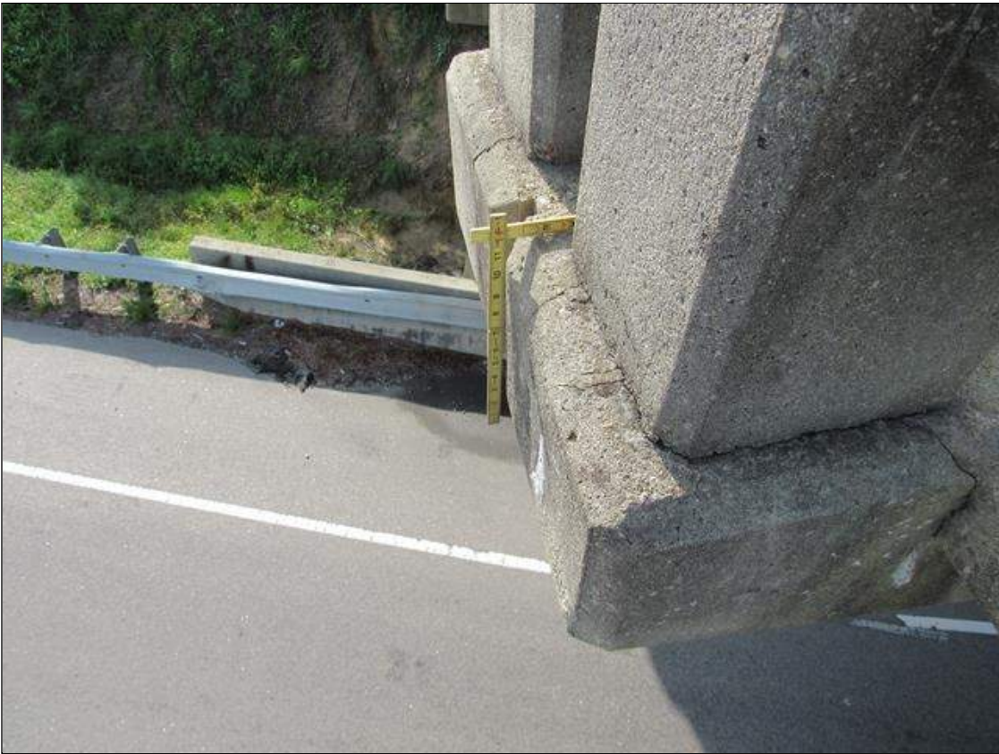
Span 3 Left Bridge Rail: (4) VERTICAL CRACKS UP TO 11 INCH LONG X 1/32 INCH WIDE, SOME WITH EFFLORESCENCE, IN 5TH SUPPORT BLOCK FROM NEAR END
